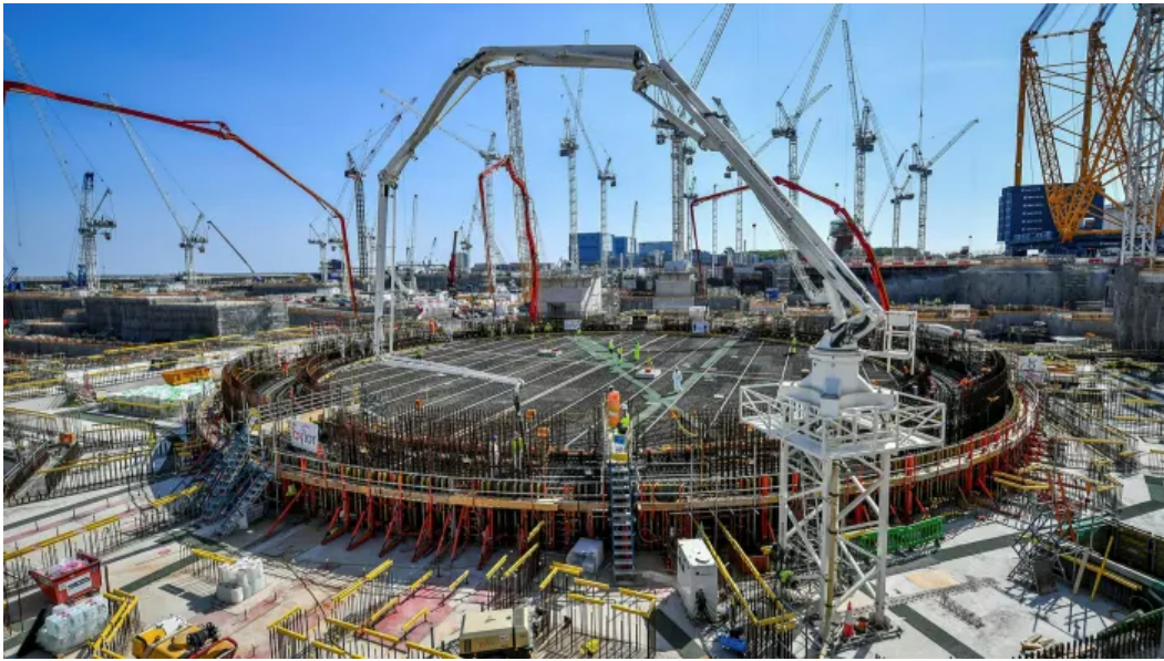
Hinkley Point C is under construction in Somerset © Ben Birchall/PA
